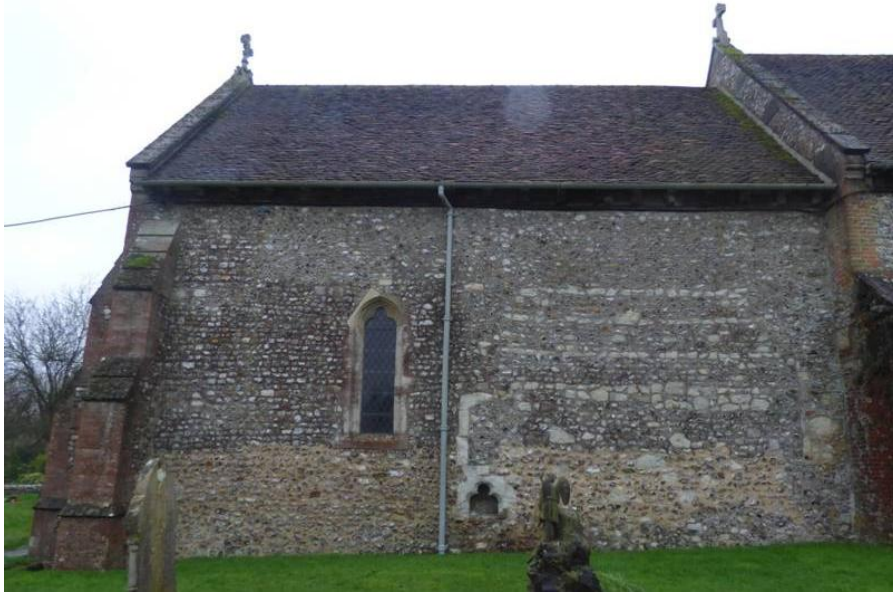
Bishop's Sutton, Hants: lancet replaced by larger window; this window blocked for north building (sacristy/chantry); building demolished.
