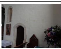
Stoke by Clare: three joist stubs of a possible organ gallery in the north wall of the chancel over and to the right of the sacristy doorway. On the upper left, the access to a passage to this gallery.
